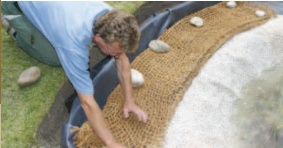
Application example: Embankment mat
