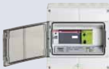
Electronic water level control 1
