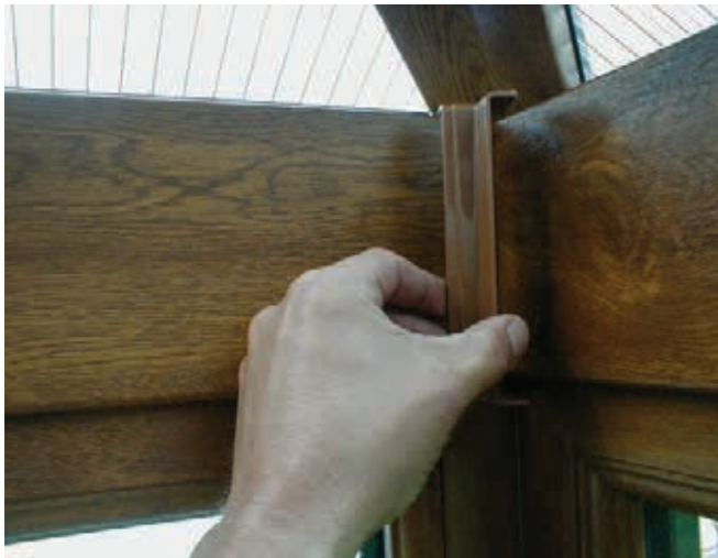
28) Fit the Trim to the Joint between the two Ring Beam Internal Trims. Repeat this process for all other Joints.
