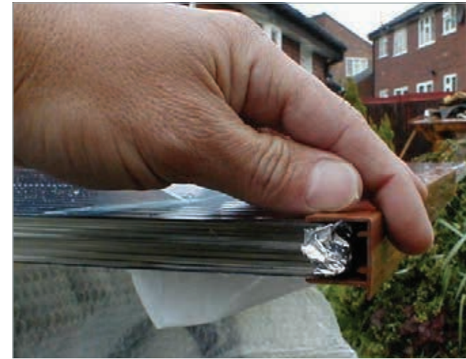
13) Fit the Glazing End Trim to the Glazing. If using Polycarbonate, peel back the protective film to enable the fitting of the End Trim. Seal End Trim using a suitable silicone sealant.
