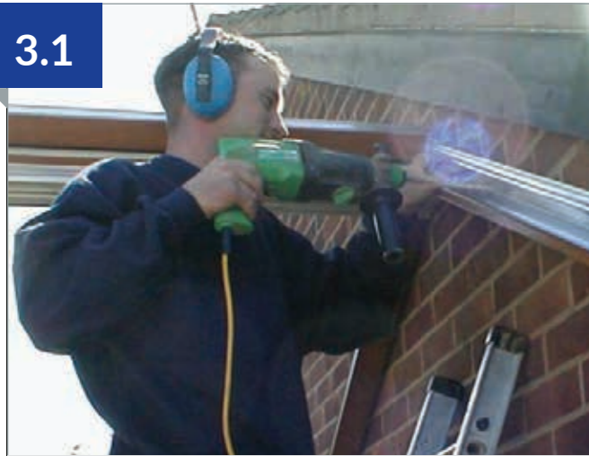
9) Fix the Gable Rafters to the Wall using appropriate fixings, minimum 3 Places per Rafter.
