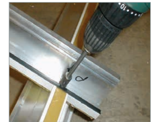
2) Place the Jack Rafter into position, locating the Jack Rafter Bar onto the Jack Rafter Fixing and onto the Double Studs at the Ring Beam End. Tighten all nuts.
